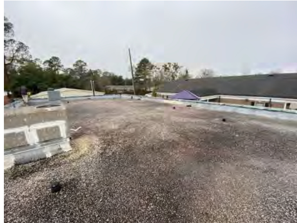
BUILDING M300 B1 PHOTO # 6
