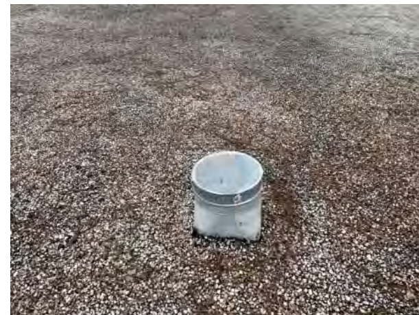
BUILDING M700 PHOTO # 12
