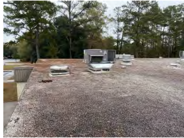
BUILDING M700 PHOTO # 2
