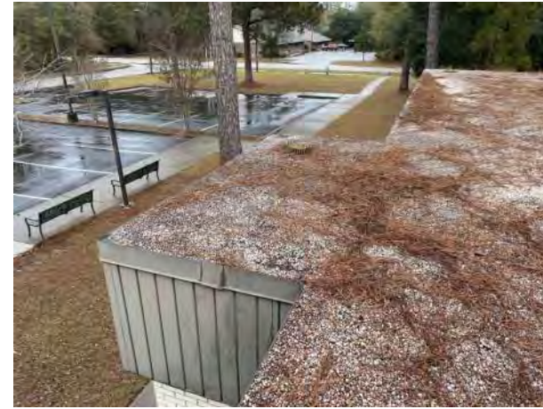
BUILDING M700 PHOTO # 4
