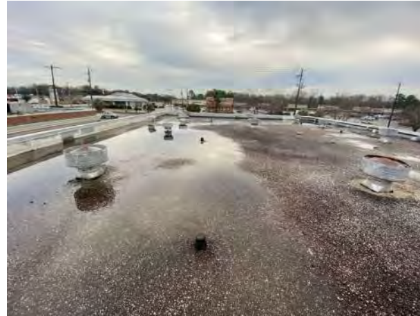
BUILDING M300 A2 PHOTO # 19
