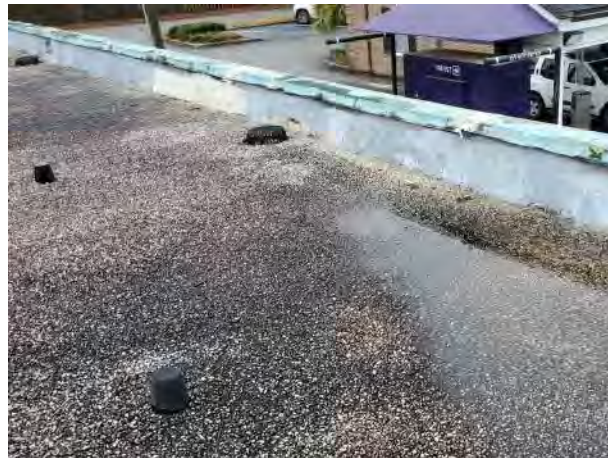
BUILDING M300 B1 PHOTO # 10
