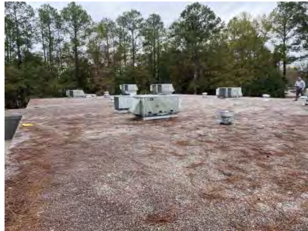
BUILDING M700 PHOTO # 5
