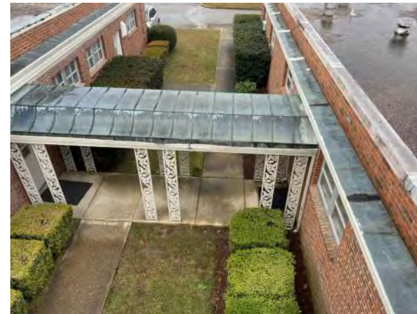
BUILDING M300 B1 PHOTO # 12
