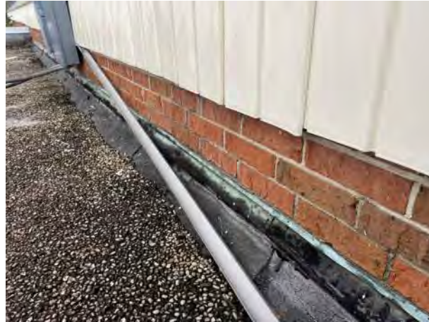
BUILDING M300 A2 PHOTO # 18
