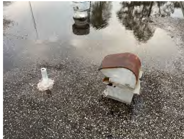
BUILDING M300 A2 PHOTO # 23
