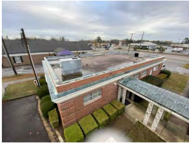
BUILDING M300 B1 PHOTO # 1
