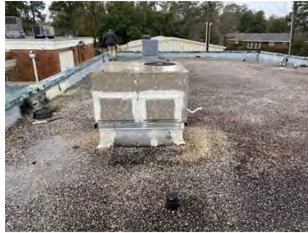
BUILDING M300 B1 PHOTO # 3
