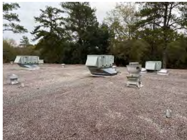
BUILDING M700 PHOTO # 9
