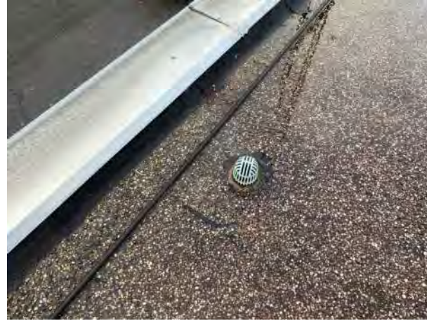
BUILDING M300 A1 PHOTO # 3
