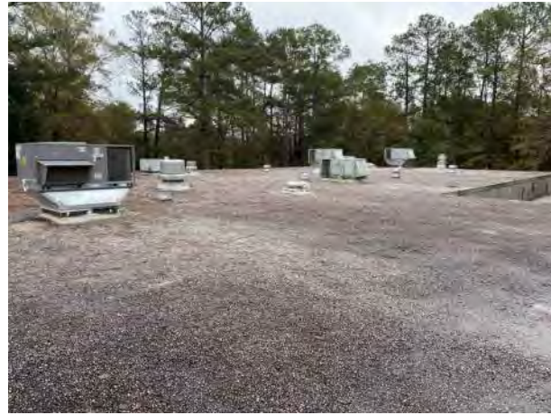
BUILDING M700 PHOTO # 1
