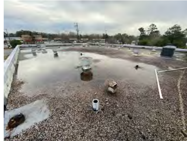
BUILDING M300 A2 PHOTO # 20
