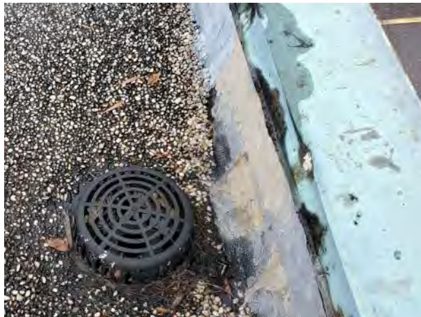
BUILDING M300 B1 PHOTO # 9
