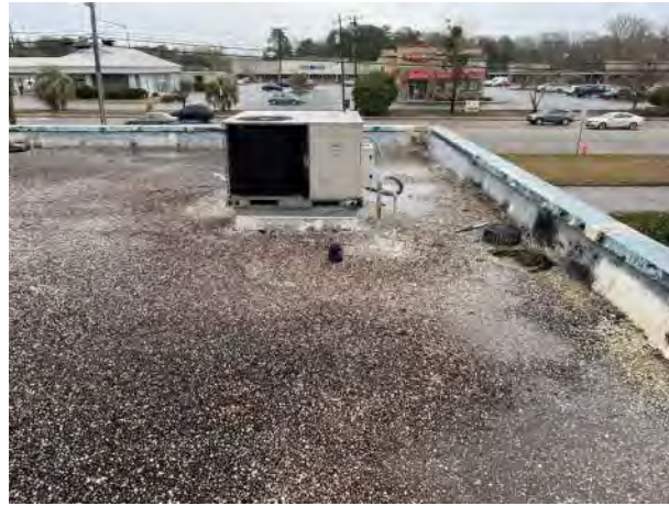
BUILDING M300 B1 PHOTO # 2
