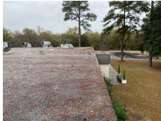
BUILDING M700 PHOTO # 6
