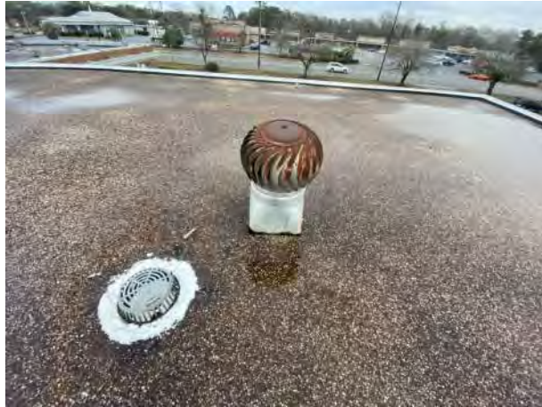
BUILDING M300 A1 PHOTO # 5
