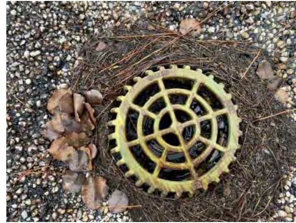
BUILDING M700 PHOTO # 3
