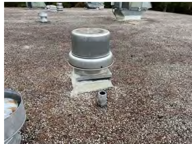
BUILDING M700 PHOTO # 11
