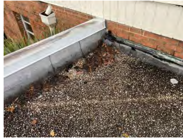
BUILDING M300 A2 PHOTO # 16
