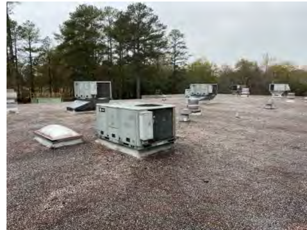
BUILDING M700 PHOTO # 7
