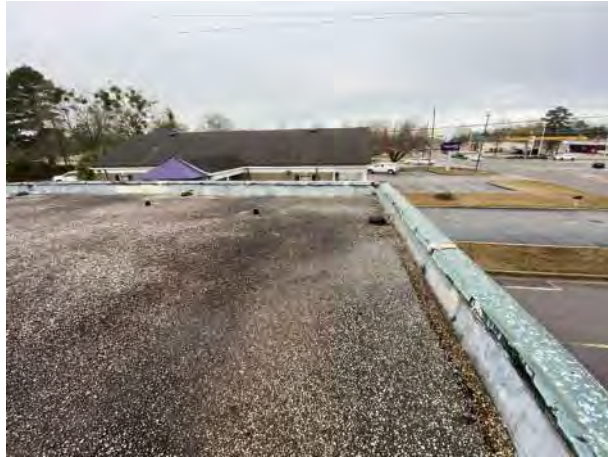
BUILDING M300 B1 PHOTO # 5
