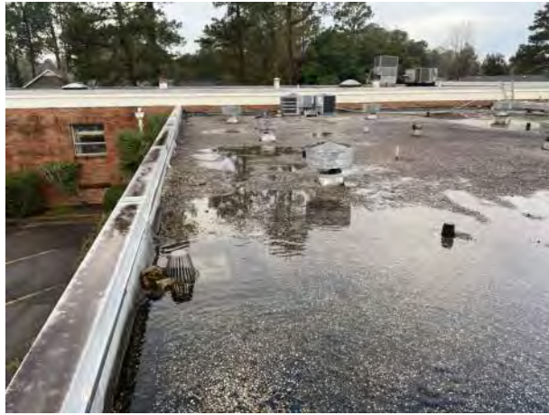
BUILDING M300 A2 PHOTO # 13
