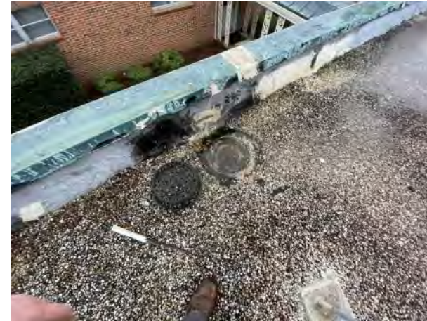
BUILDING M300 B1 PHOTO # 8
