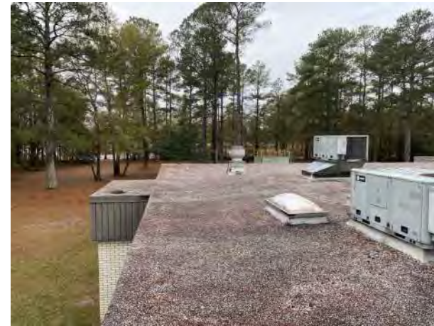
BUILDING M700 PHOTO # 8
