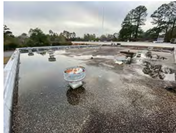
BUILDING M300 A2 PHOTO # 24
