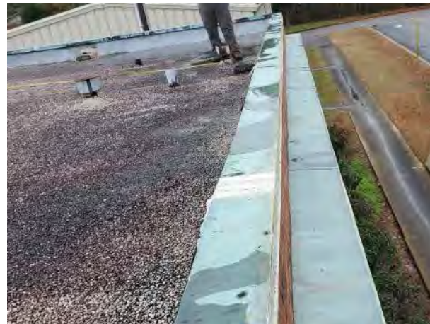
BUILDING M300 B1 PHOTO # 11
