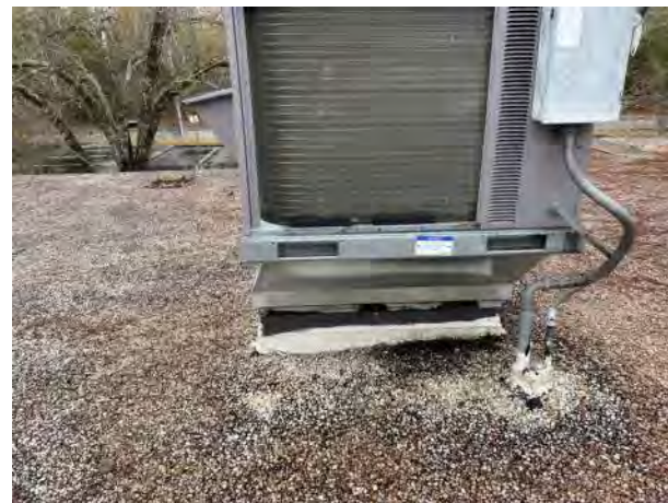
BUILDING M700 PHOTO # 10
