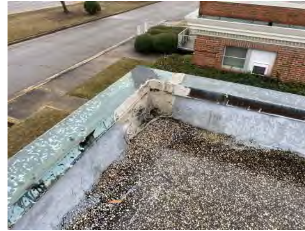
BUILDING M300 B1 PHOTO # 4
