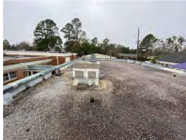
BUILDING M300 B1 PHOTO # 7
